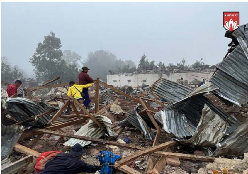
The MDY-PDF's POW detention facility destroyed in the junta airstrike. (Photo- MDY PDF)
