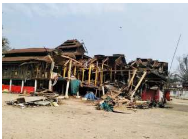
Kyaung Kham temple damaged by SAC shell
