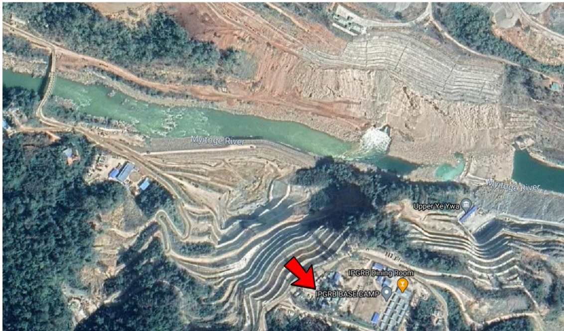
Google satellite image of Upper Yewa dam-site with "IPGRB BASE CAMP" label
