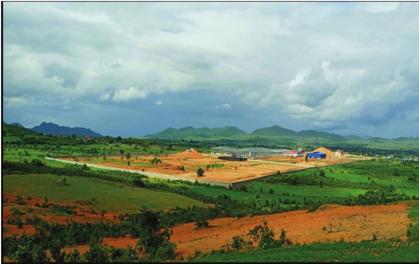
Mineral refinery construction at Nwa La Boe (Credit: KMIW)
