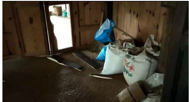
Villager's house door broken by Burma Army
